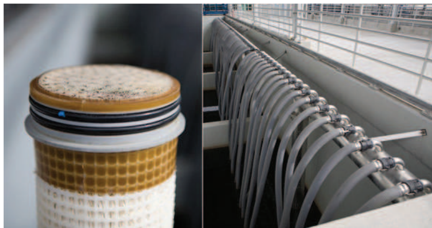
Water Factory 21- 326 ML/d (26 x Memcor® CS608)
